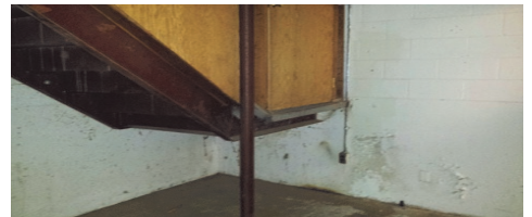
Fall Hazard (no steps) (4ft drop off)
